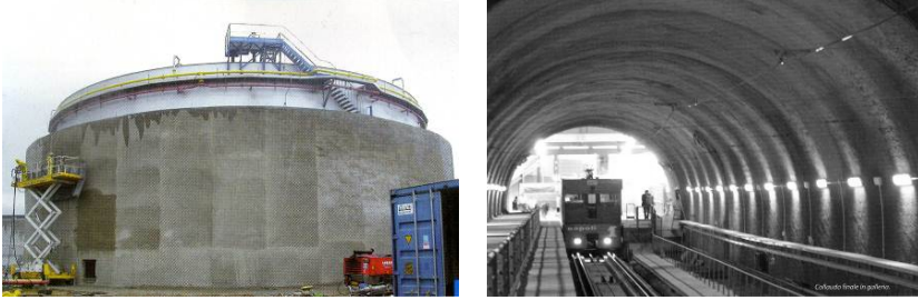
Fig. 1. Structural use of shotcrete (left) in a cylindrical shield for the protection of an oil tank (France, Atlantic Coast); and use of sprayed mortar (right) for water-proofing the lining of an urban tunnel (Italy, Naples), both from Realtà Mapei, V. 96, N.9, 2009.
