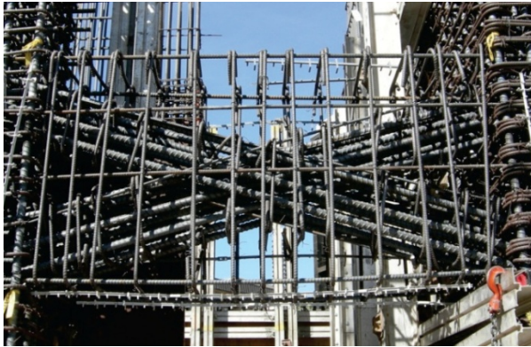
Fig. 1. Reinforcement detailing in diagonally reinforced coupling beam
